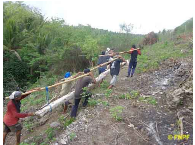
The volunteers and local villagers hauling logs for building the new center.
